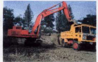
Excavation equipment from Auroville's Water Harvest service deepening Annapurna's pond
